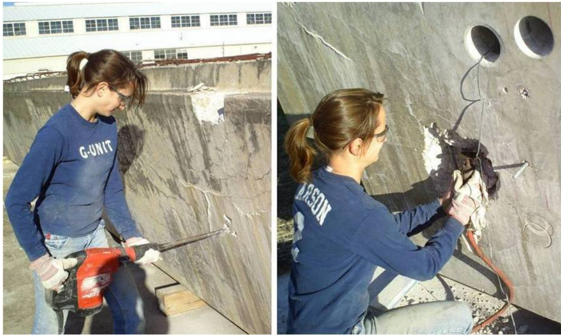
Figure 5-11: Exposing and Cutting the Transverse Reinforcement
