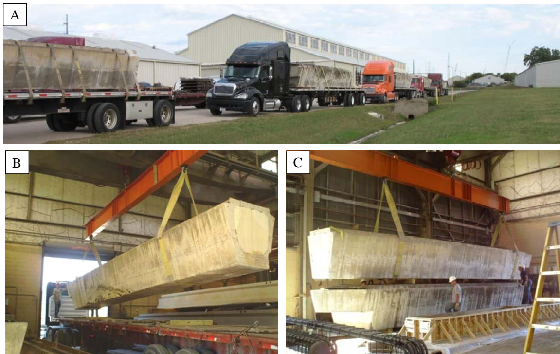
Figure 3-2: Arrival of Beam Segments from Mesa Precast Yard
