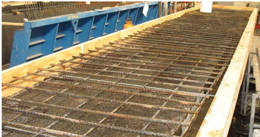
Figure 3-25: Formwork and Rebar for the Topping Slab
