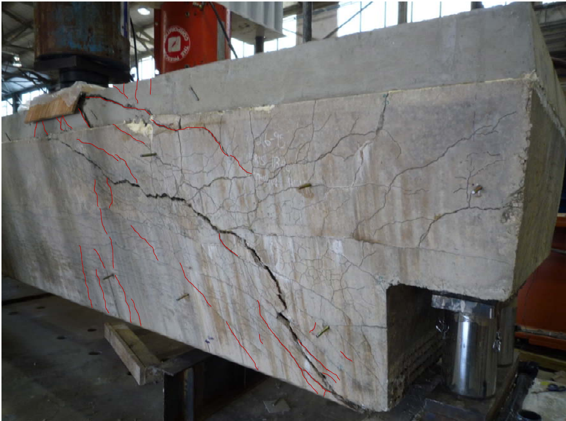
(C) Post-Failure Growth of ASR/DEF Cracks
