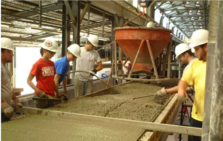
Figure 3-26: Casting the Deck of Segment H-II
