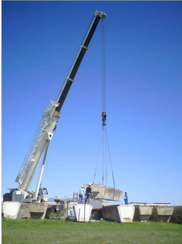
Figure 3-3: Handling of Beam Segments with a Mobile Crane
