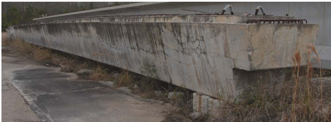
Figure 3-1: Trapezoidal Box Beam Storage at Mesa Precast Yard
